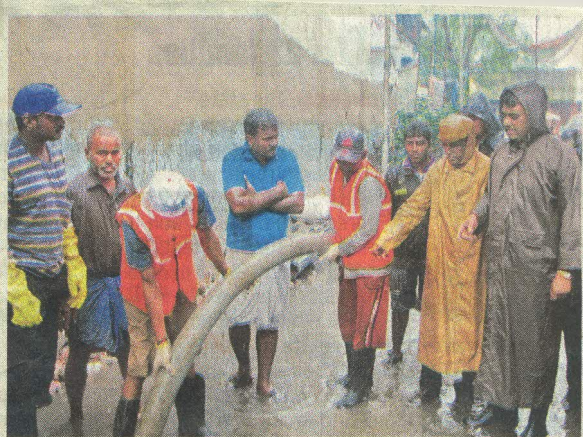
Chennai Metro Water MD Chandramohan (extreme right) getting stagnant water removed
